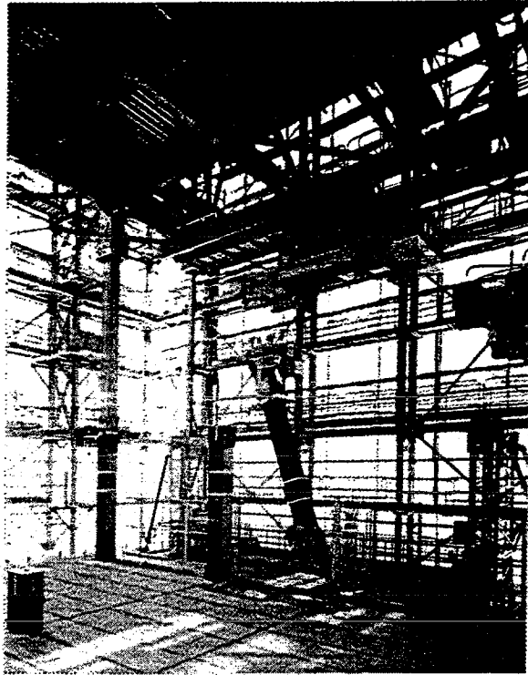
photo. 3 Steel column erection with SCF Crane
