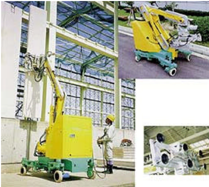
Figure 7: This multi-jointed handling robot assists in the installation of heavy exterior and interior materials (FUJITA Japan).
