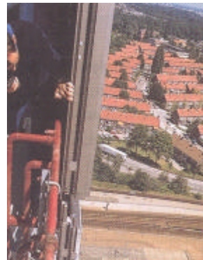
5. Wall panels are assembled.
