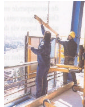
4. Wall panels are connected to the tower crane.
