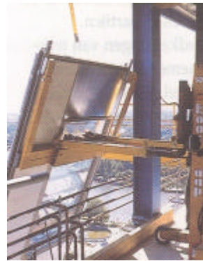
3. Wall panels are moved outside.
