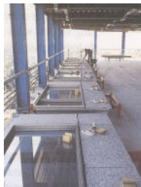
2. Wall panel depot on the floor where the panels will be installed.
