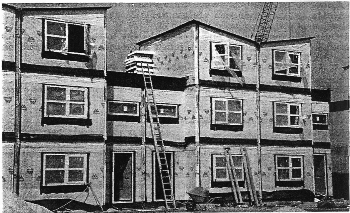
Figure 8. Permanent houses in construction.
